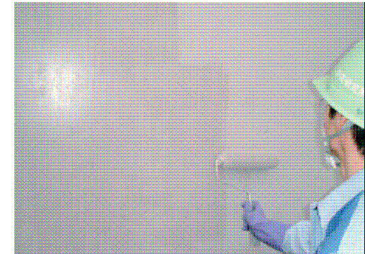
Taiheiyo ST-coating material containing photocatalytic \text{TiO}_2
